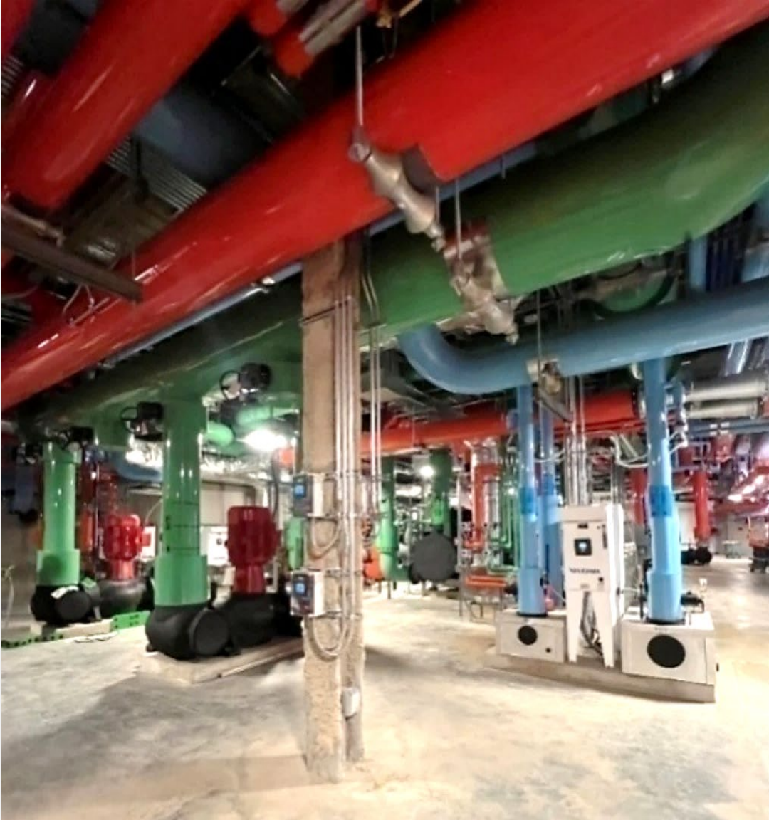
Picture 1 Color Coded Piping Corresponding to Water Temperature Used in Geothermal System 2025
